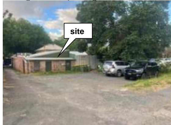
Figure 2.3: Informal car parking area at rear of the site
