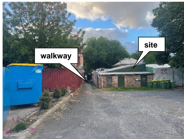
Figure 2.7: Laneway looking north from Furmston Lane
